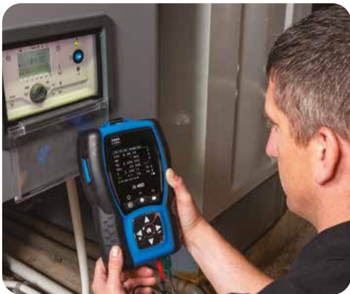
Confirm boiler safety & efficiency
